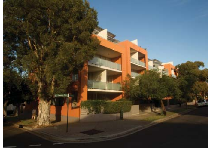
Corner of Dunning Avenue and Queens Road
