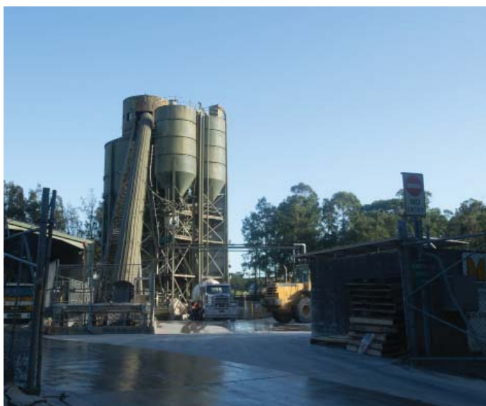
Concrete Batching Plant
