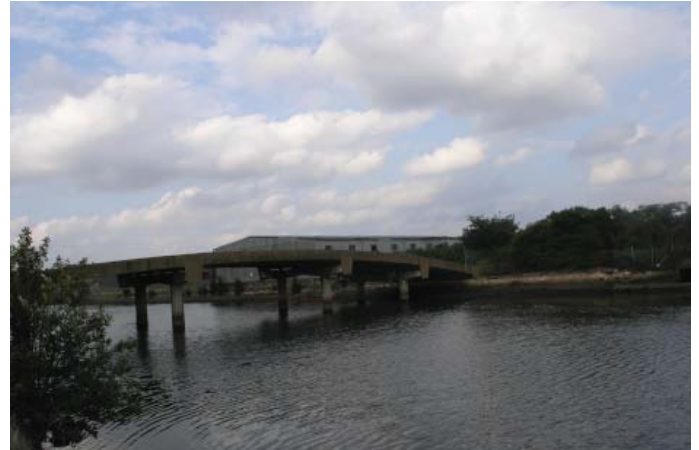
Alexandra Canal Vehicular Crossing - Gardeners Road
